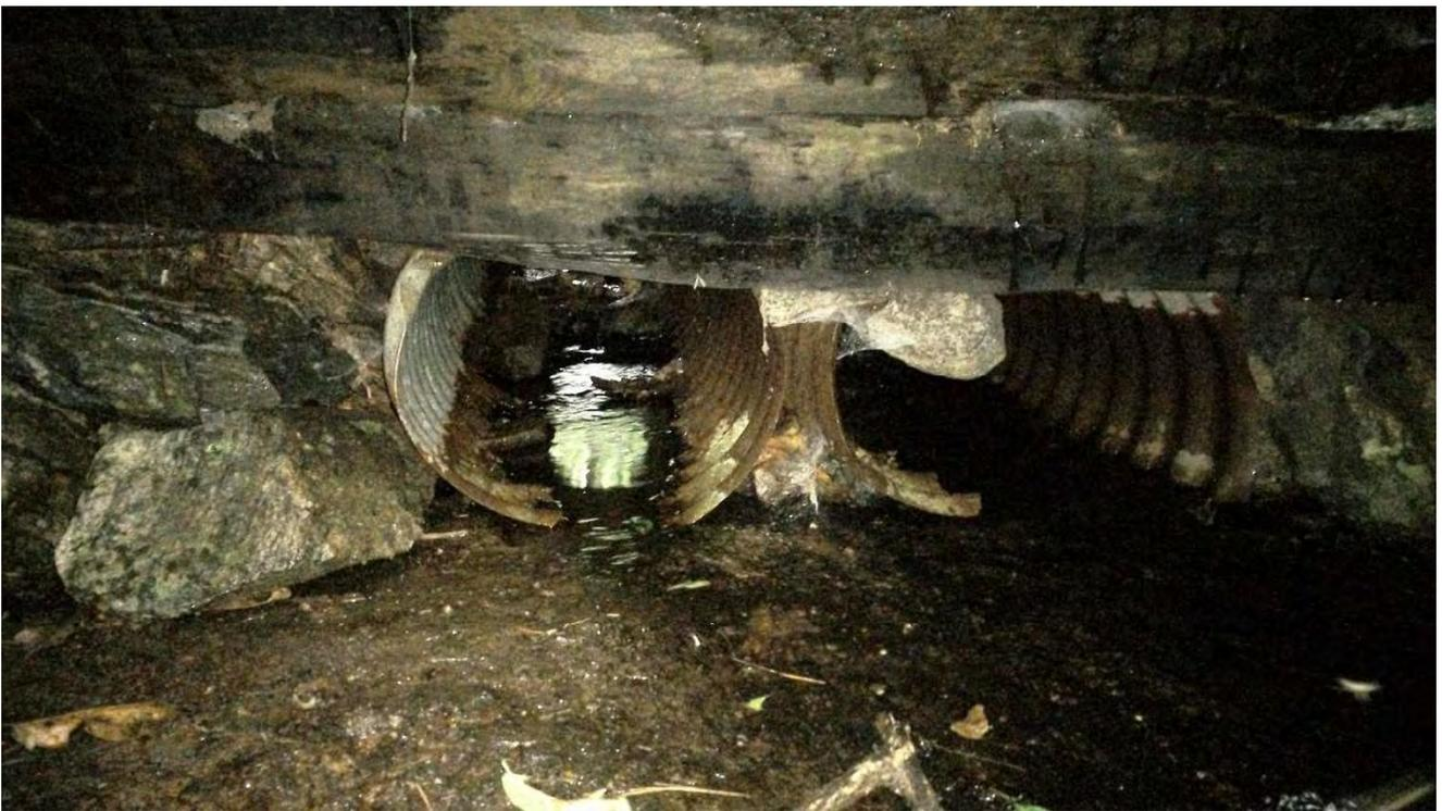
**Photograph 14: Culverts under trail at west branch stream crossing**
